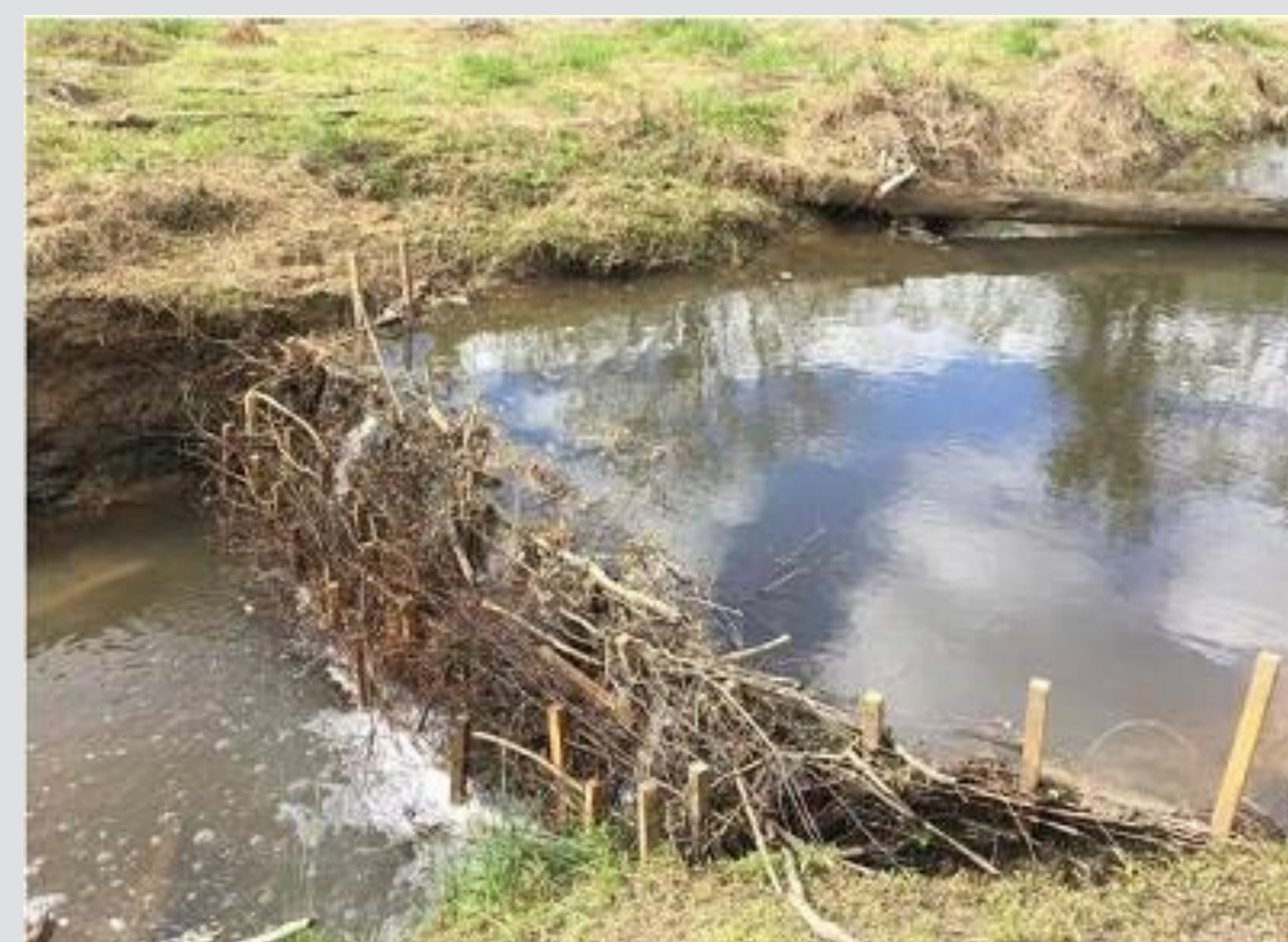
Beaver dam analog (BDA) constructed near Yates Mill Pond by Adam Lee (2017).
